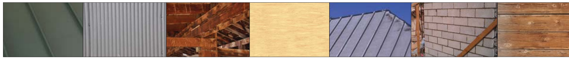
forest green standing seam roofing (existing structures) reclaimed corrugated steel cladding from existing siding original barn structure (typical) plywood interior finish of SIPS panels zinc standing seam roofing (spine) concrete block wall (spine) reclaimed wood for entry cavity wall screen
