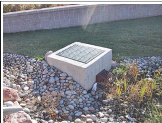
Photo 3: Detention pond outlet with trash/safety racks
