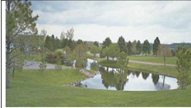
Photo 7: Retention pond with various safety provisions, including mild sideslopes and shallow water around full pond perimeter
