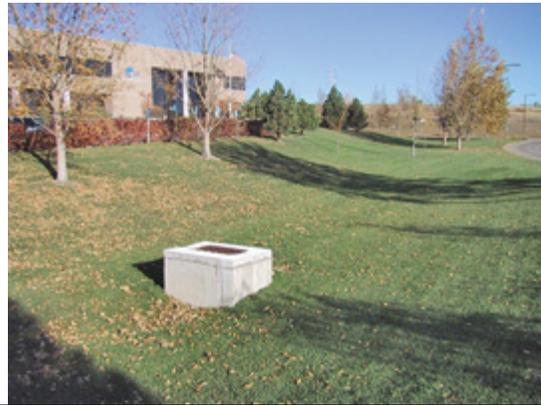
Photo 4: Detention pond with safe outlet, placed mid-pond, with mild sideslopes and good visibility from office building
