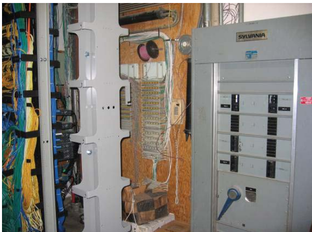
Figure 3.2.3a – TR Room with Electrical Equipment
