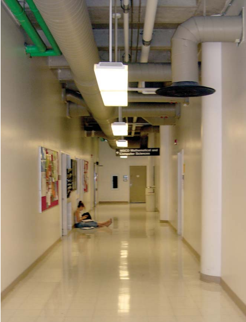
Figure 3.2.1a – Typical corridor of existing Science building
