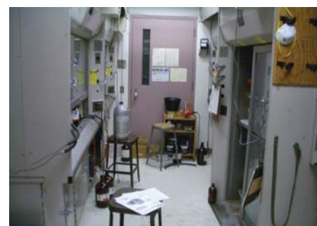
Figure 3.2.2a – (upper left) Existing MSCD Chemistry Instrumental Analysis Laboratory. Figure 3.2.2b – Corrosion of fume hood duct in UCDHSC Chemistry Research Lab Figure 3.2.2c – (bottom) Existing UCDHSC Chemistry Research Lab
