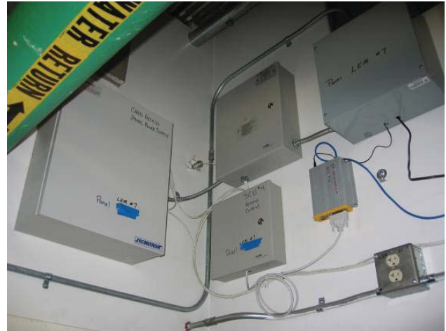
Figure 3.2.3g – Access Control System Components
