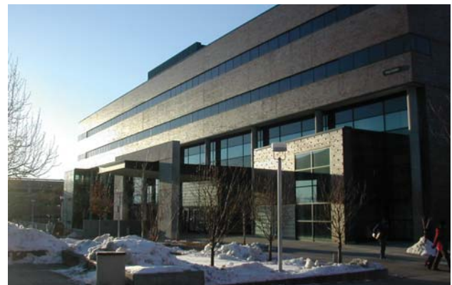
Figure 3.1b – North Classroom building
