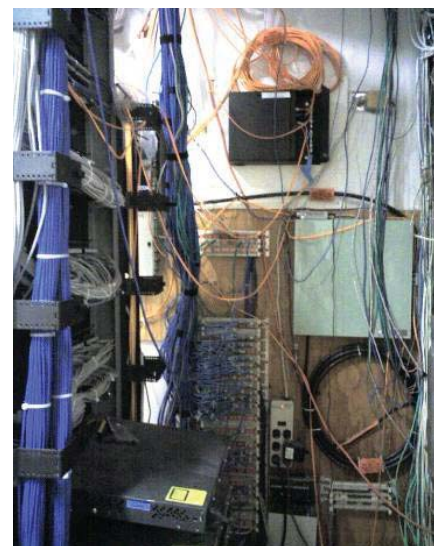
Figure 3.2.3c - Various Termination Blocks and Panels
