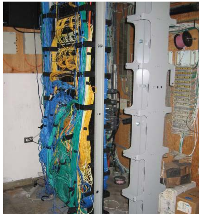
Figure 3.2.3b – TR Room with Heavily Loaded Equipment Rack
