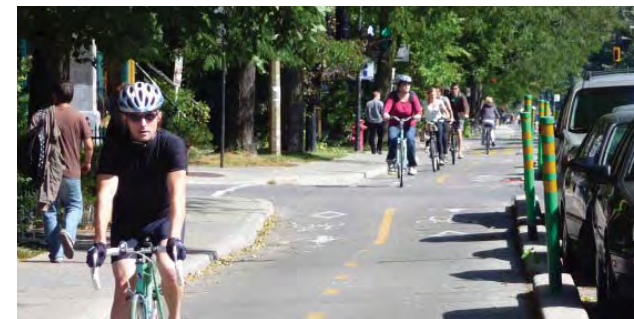
Figure 6.6: Bi-directional bike lane example with buffer and on-street parking, Montreal, Canada
