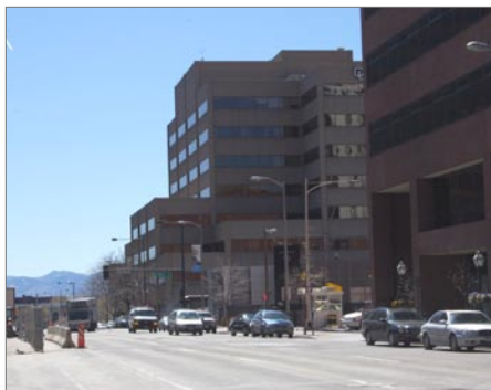
Dravo Building View from 15th St. & Lawrence St.
