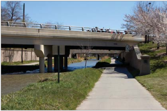
View of Cherry Creek Trail below grade
