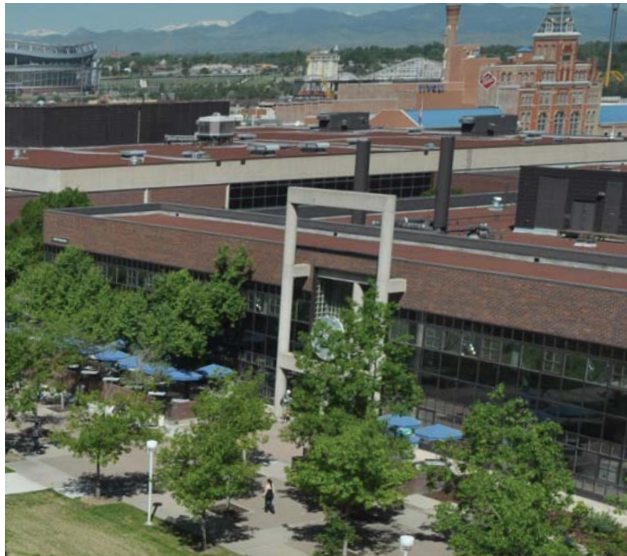
Existing North Classroom roof.
