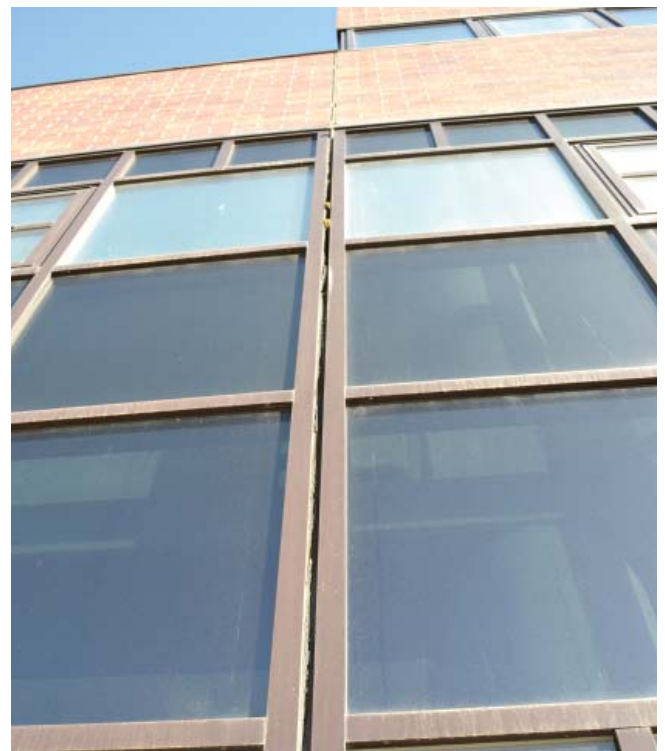
Failing window seal.
