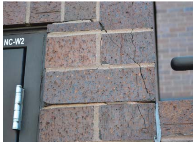
Exterior cracking around door.
