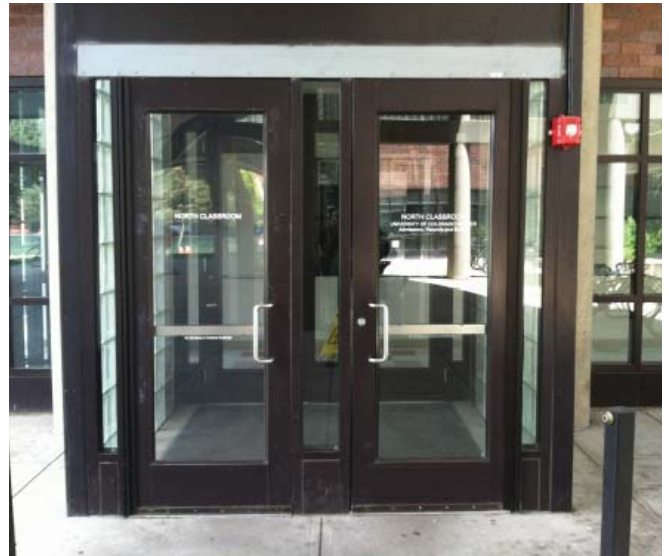
Exterior doors that require ADA upgrades.
