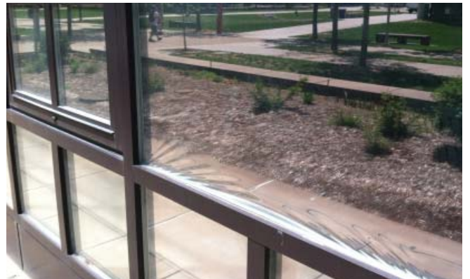
Warped window film.
