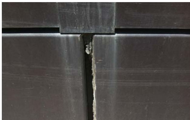
Failing exterior sealant.
