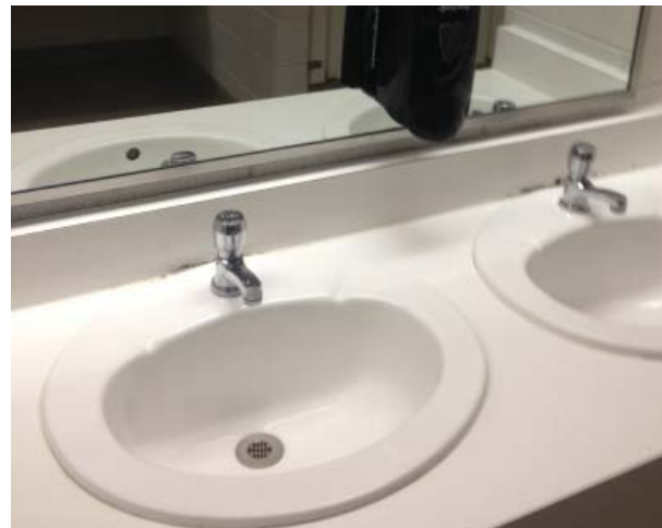
Original North Classroom bathroom fixtures.
