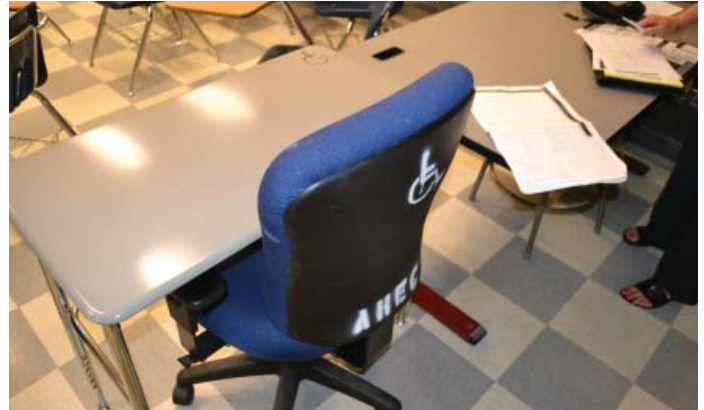
Poor ADA accessibility.
