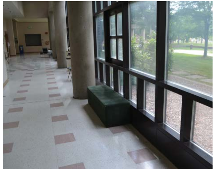
Green carpet block seating does not provide any work area.
