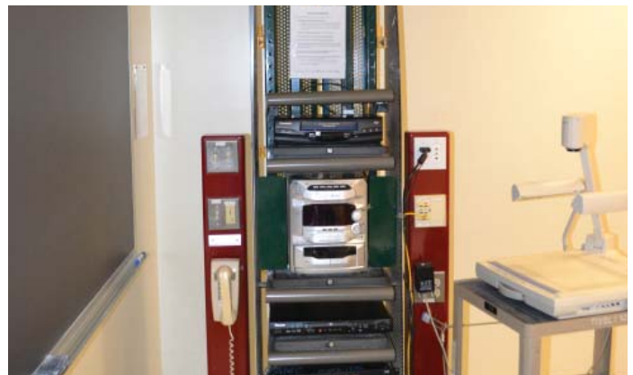
Existing classroom with out-of-date technology.
