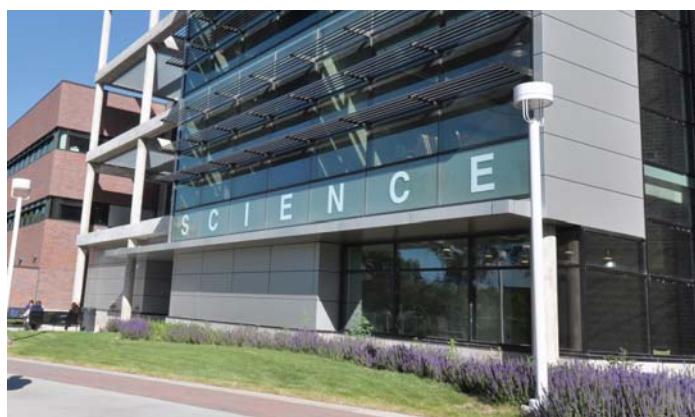
The Science Building.
