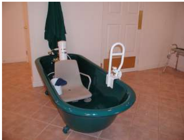
Tub Handrails / Tub Seat
