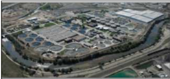
Wastewater Treatment Plant
